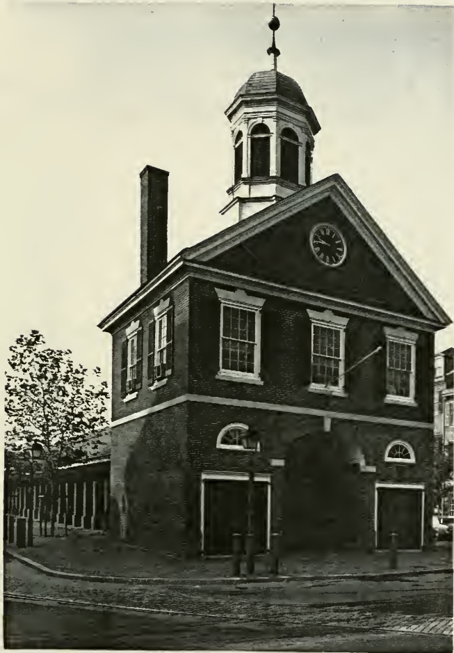
Second Street Market, front elevation, Head House
